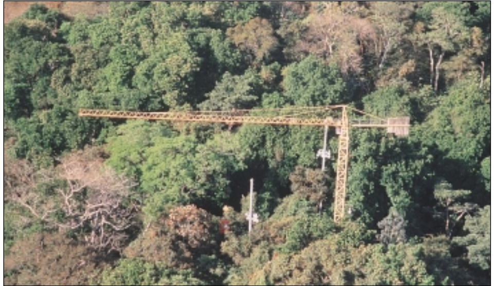
The Smithsonian Tropical Research Institute (STRI) has erected a construction crane in the Metropolitan national park of Panama. The crane is 42 m tall and has a horizontal boom of 51 m, thus, it facilitates the study of approximately 0.8 ha of tropical forest. The crane provides access to the outer branches of all levels of the forest, allowing species to be studied in their natural habitats.
